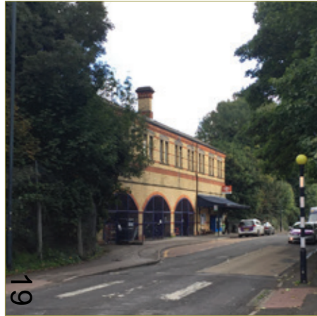
Maidenhead Railway Station access off Shoppenhangers Road
